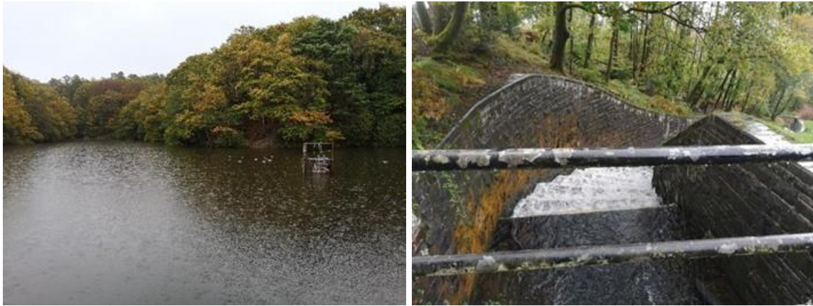
A range of attractive and stunning water features (top left cascade and other are the reservoir and overflow)
